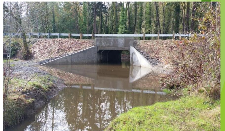
Figure 3: Harper Creek after the removal of a culvert and addition of a bridge to allow adequate water flow in and out of the estuary. This is predicted to allow salmon access to the Kitsap County local streams, which in turn may increase salmon populations and biodiversity. (<https://pugetsoundblogs.com/waterways/2016/11/09/harper-estuary-project-gets-started-following-years-of-discussion/>)
